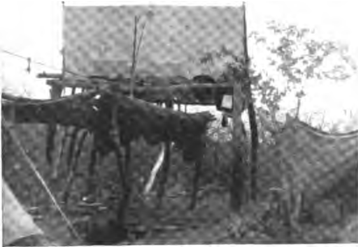
“FIVE SIKH CARPENTERS HAD MADE A STAGING.”
